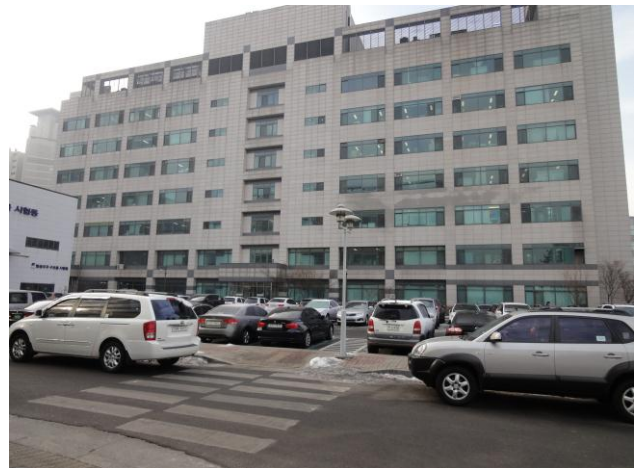
Fig. 1 CAPST is inside this building
